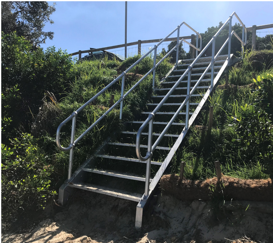
Beach access stairs - Hastings Point
