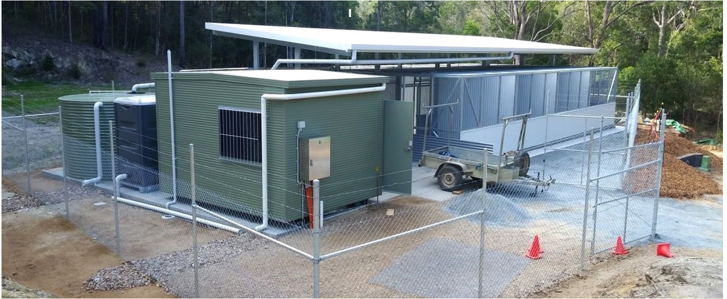
TCKRH construction complete Jan 2021
